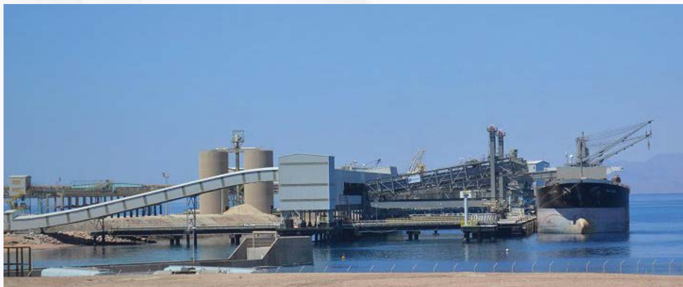
The new phosphate export terminal, one of Jordan Phosphate Mines Company PLC's investments.
